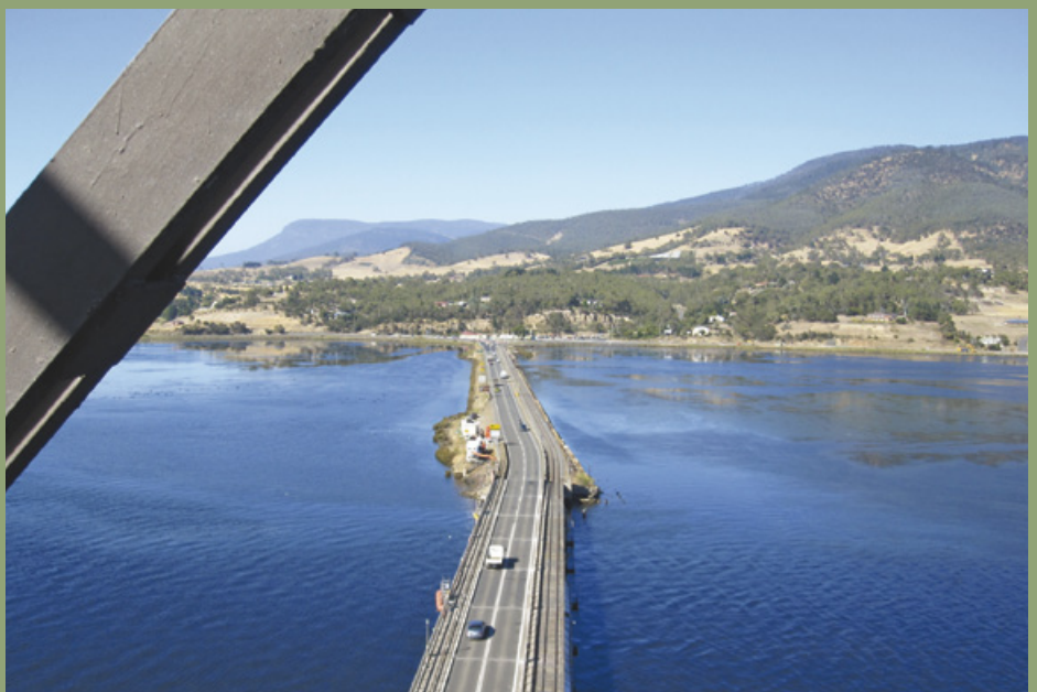
View from the Bridgewater Bridge
