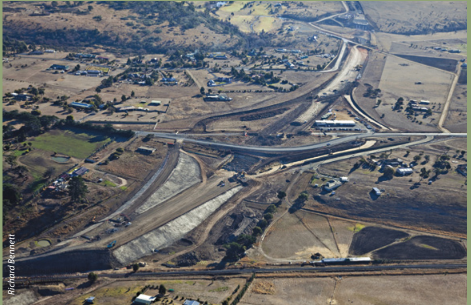
Tea Tree Road Interchange looking north
