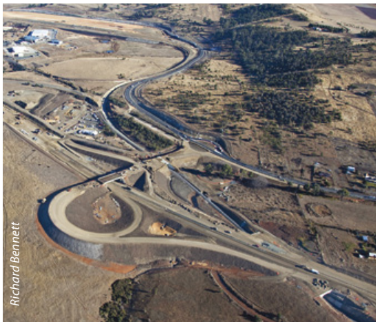
Brighton Interchange looking southbound
