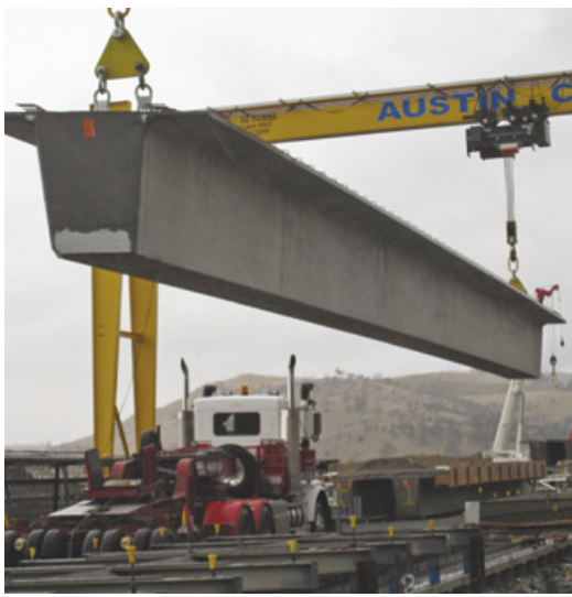
Pre-cast yard - Rifle Range Road beam
