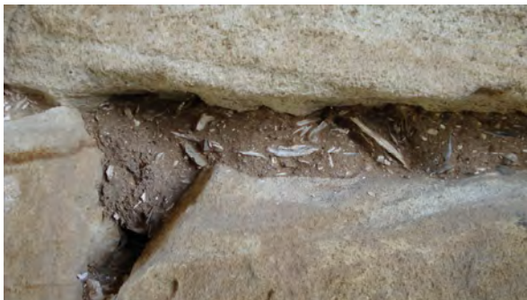
Coarse shell mortar
