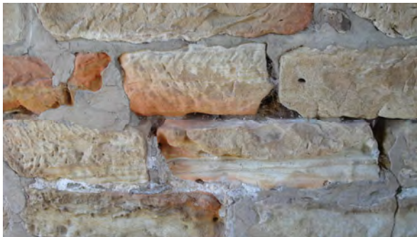
Degree of stone decay and loss of mortar
