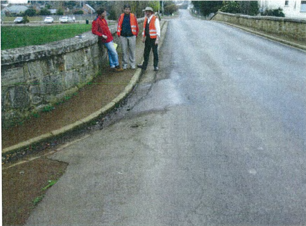
Photo 1 Note water ingress causing pavement failure adjacent to sensor location 1.
