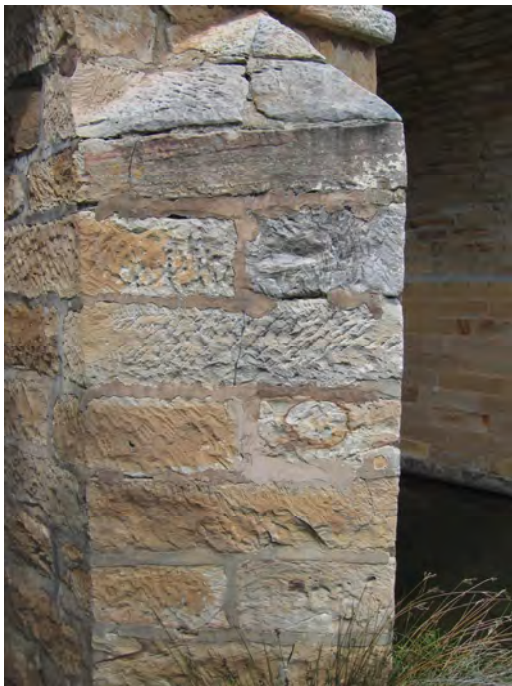
Cracks eastern pier
