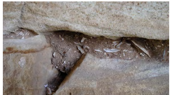
Salt efflorescence on mortar joints and stonework
