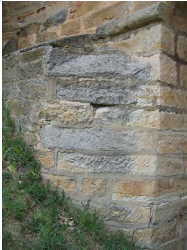
Cracks in north east abutment
