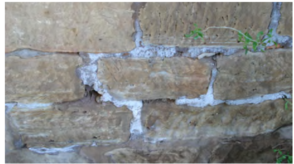
Salt efflorescence on mortar joints and stonework
