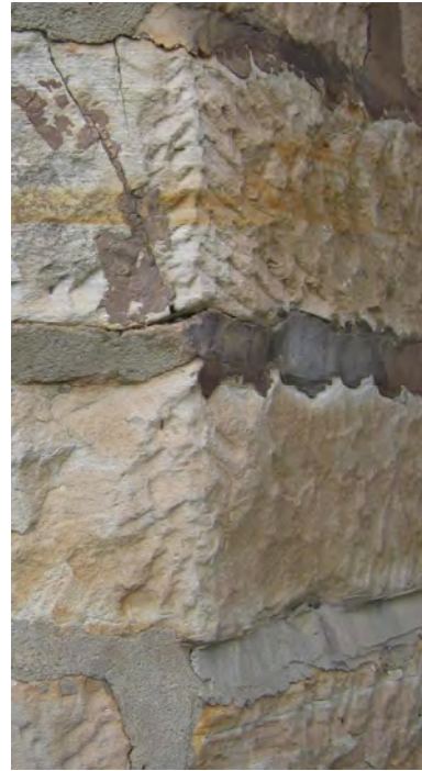
Detail, cracks in north east abutment
