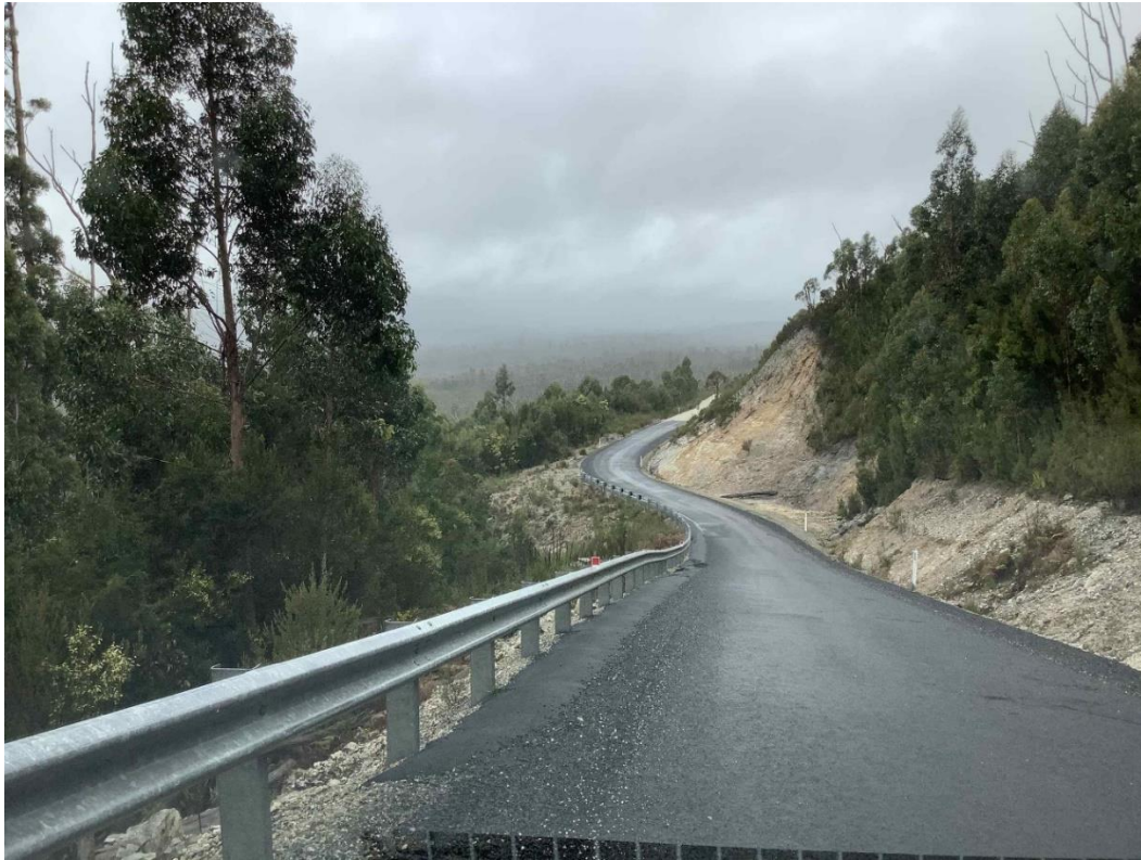
Figure 5: Ch 11.2 km Sealed section
