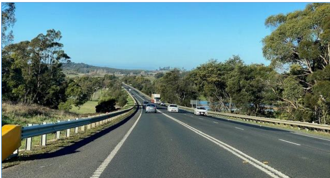
Figure 6.1: Example of narrow shoulder near Deloraine
