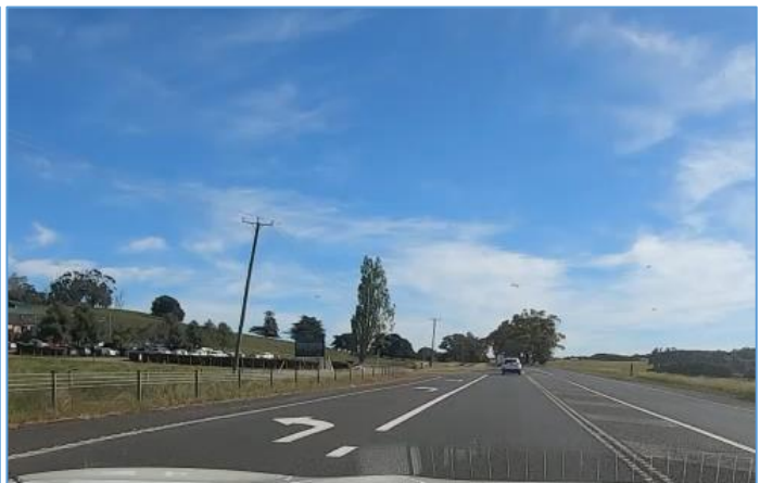
Bass Highway, at entrance to Ashgrove Cheese Dairy entrance with short deceleration lane
