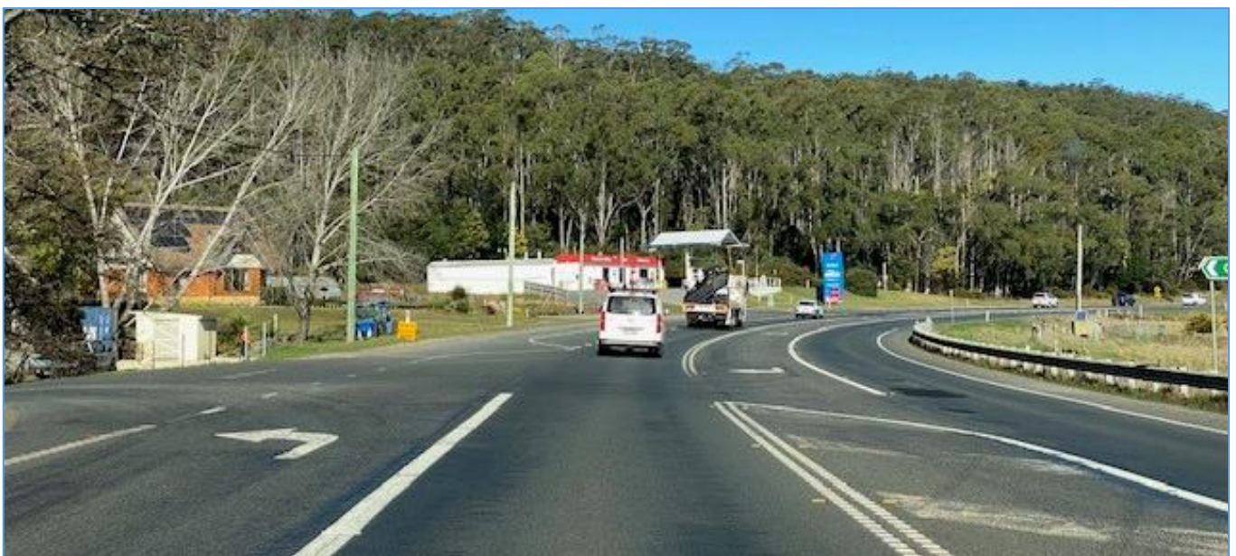
Figure 4.12: Bass Highway at Parkham Road travelling south
