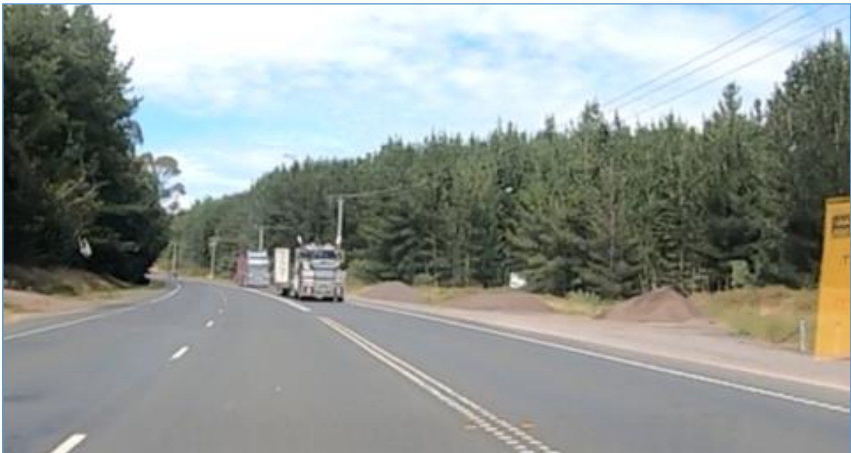
Figure 3.1: Trucks on the highway
