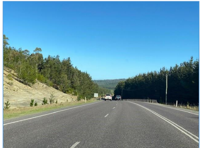
Bass Highway, Parramatta Creek, eastbound
