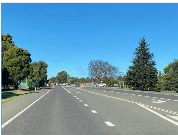
Bass Highway, in Latrobe, looking east
