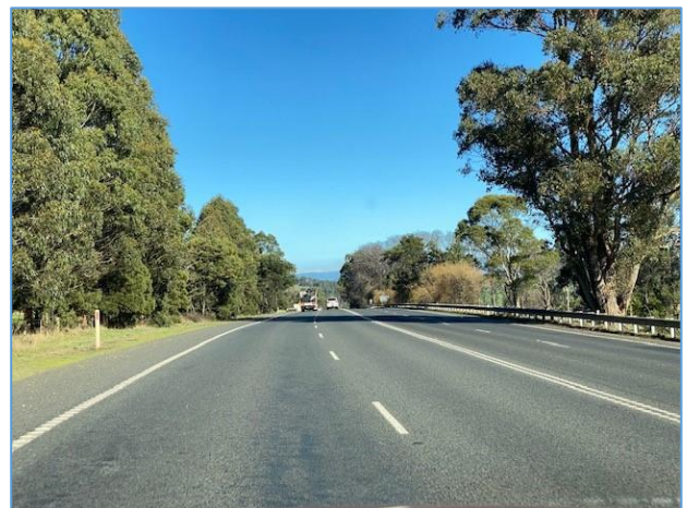
Bass Highway, near Elizabeth Town, looking east
