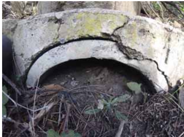
Photo Inlet – Upstream outlet 400mm from culvert inlet
