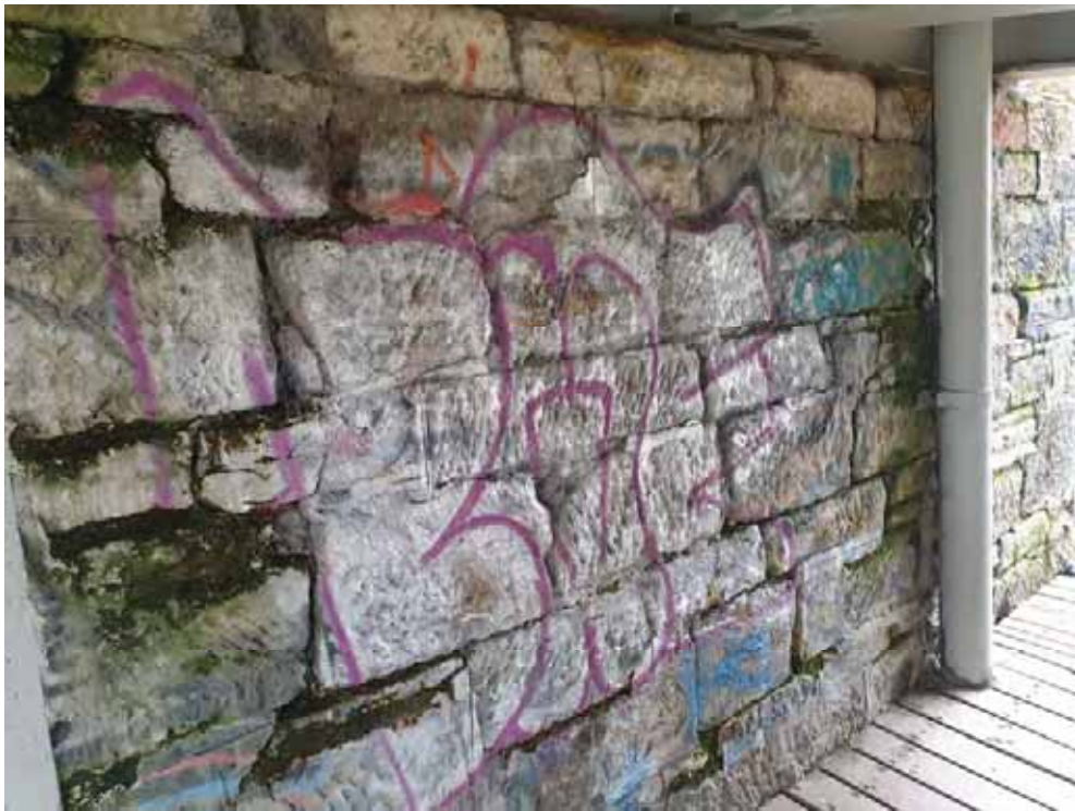
Deteriorated sandstone wall at Abutment 1
