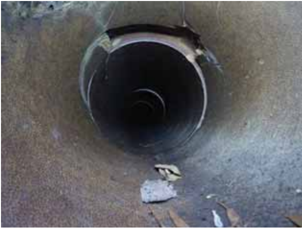
Photo Inlet – view towards outlet
