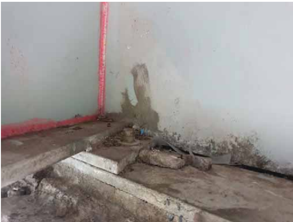
Figure 8 Inadequate bolts at the bearings (typical)
