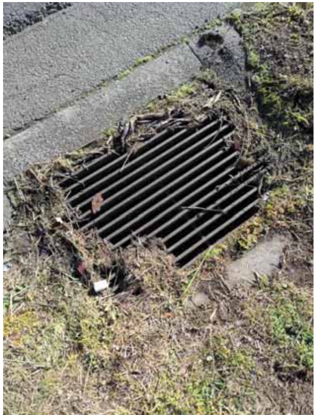
Photo Inlet – pit adjacent to the footpath appears to flow towards pit along the road
