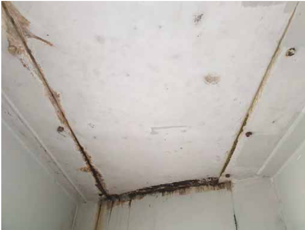
Figure 7 Deteriorated bolts connecting the girders to the deck
