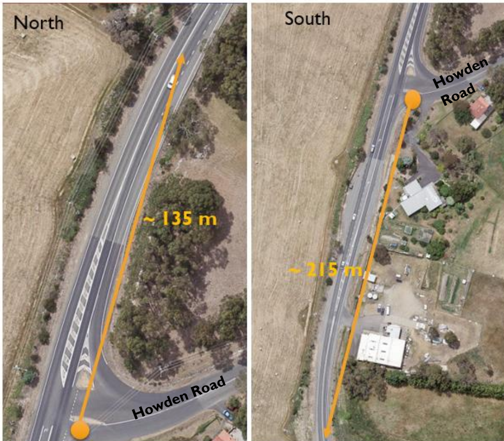
Figure 31 Howden Road intersection – Available sight distance
