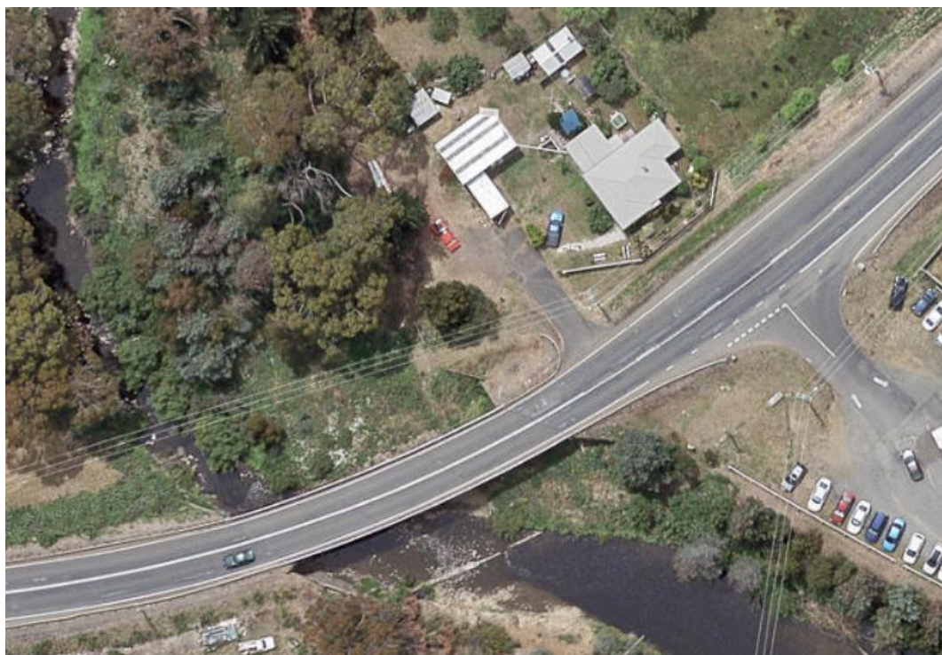
Figure 32 North West Bay River bridge
