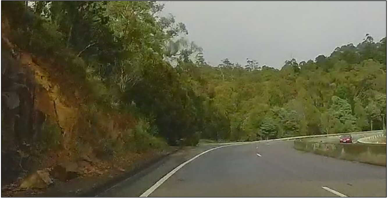
Figure 5-4 Rockfall hazard, south of Sandfly Road
