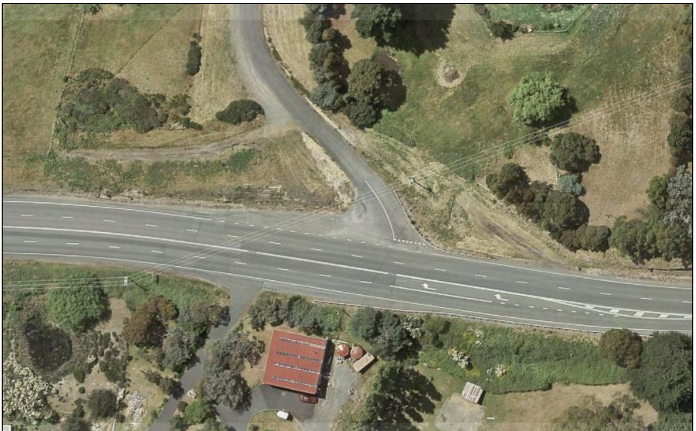
Figure 4-11 Deficient length southbound overtaking lane starting at Huon View Road
