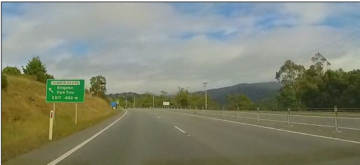
Figure 3-5 Recently upgraded section, north of Summerleas Road
