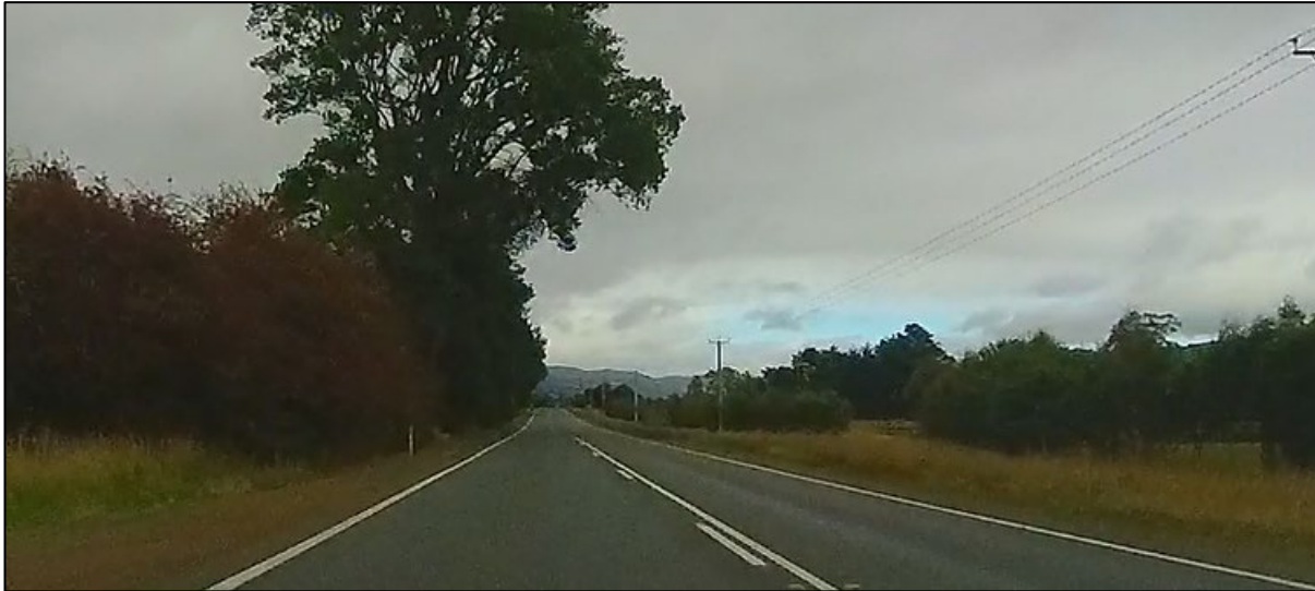
Figure 3-9 Single carriageway, south of Mountain River Road
